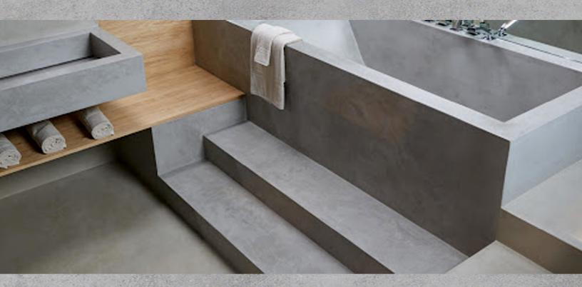
MICROCEMENT IS A TYPE OF DECORATIVE COATING USED FOR FLOORS AND WALLS. IT IS MADE FROM A COMBINATION OF CEMENT, RESINS, AND OTHER CHEMICALS. DUE TO ITS HIGH RESISTANCE AND ABILITY TO BE APPLIED ON VARIOUS SURFACES, INCLUDING CEMENT, CERAMIC, TILE, GYPSUM, PLASTIC, GLASS, METAL, STONE, AND WOOD, IT IS KNOWN AS A POPULAR OPTION IN THE CONSTRUCTION AND INTERIOR DESIGN INDUSTRY.
